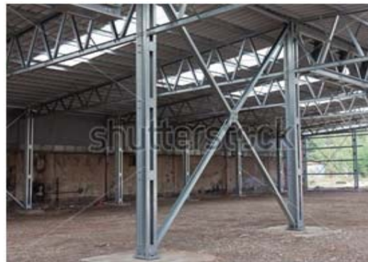
Fig: 1. Concentrically x-bracing
