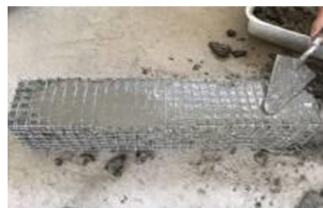
Fig 4 Retrofitting of beams
