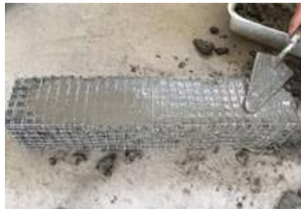
Fig 3 Retrofitting of beams
