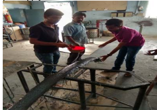
Fig(3.3.3(c)): Applying resin on carbon fiber
