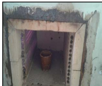
Fig 1.4.2 Heat treatment Furnace
