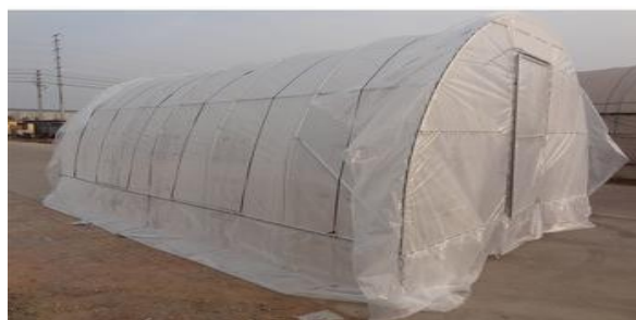
Fig.4 general construction of green house
