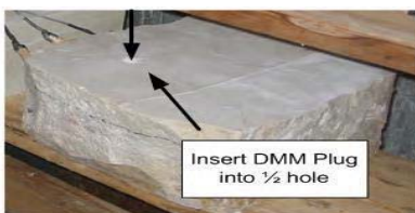
Figure: 1 Installation of EMM plug
