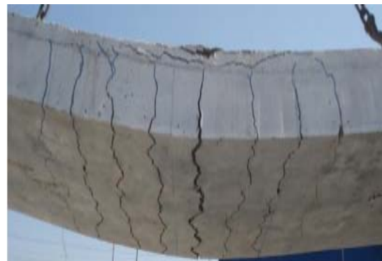
Fig. 6 Crack pattern of specimen without lacing
