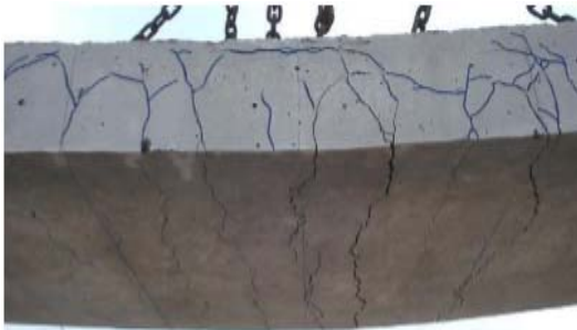
Fig. 7 Crack pattern of specimen with lacing
