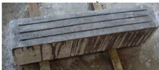
Grooves made on the surface of the concrete
