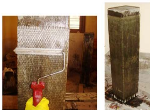
Strengthening by EBR method
