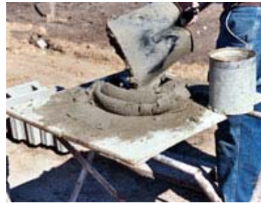
Fig 1: Retempering of concrete
