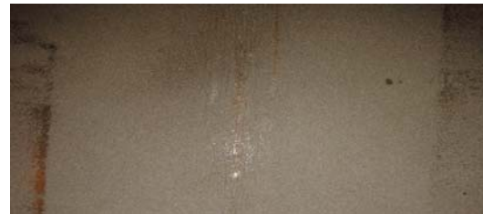
Fig.12 Crack initiation after Bend test
